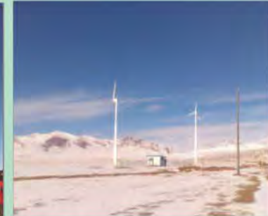
This system includes 10kw wind turbine, controller, off grid inverter, 80pcs 12V40Ah batteries and 12m hydraulic tower. In Tibet, there is no electricity in the daytime, so they need our wind turbine to supply power to them in the daytime. Until now, this system work very well.
