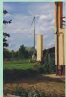
The system includes wind turbine, controller, grid-tied inverter and hydraulic tower (12m). Until now, this system work very well and can power to house use.
