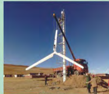
This system includes 10kw wind turbine, controller, off grid inverter, 80pcs 12V40Ah batteries and 12m hydraulic tower. In Tibet, there is no electricity in the daytime, so they need our wind turbine to supply power to them in the daytime. Until now, this system work very well.
