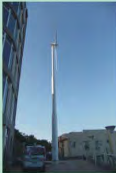
This system includes wind turbine 20kw/360v, controller, 60pcs 12v/200ah batteries, off grid inverter and hydraulic tower (18m). Until now, this system work very well and can power to hospitals continuously.
