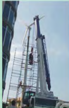
This system includes wind turbine 20kw/360v, controller, 60pcs 12v/200ah batteries, off grid inverter and hydraulic tower (18m). Until now, this system work very well and can power to hospitals continuously.
